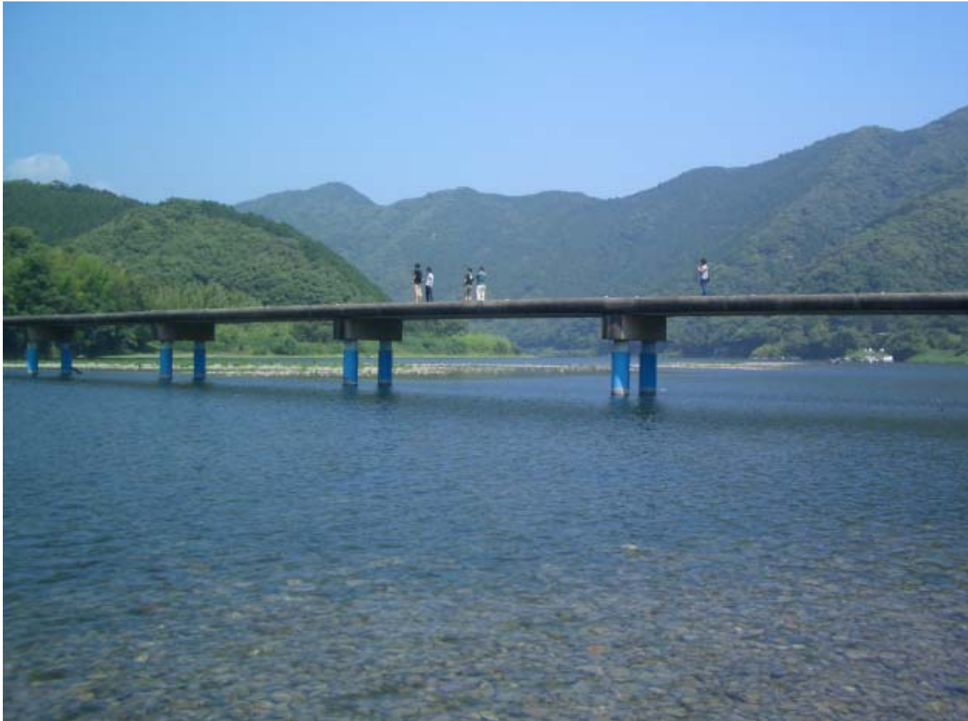
Point A: Chinka-bashi ( sinking bridge ) Width:4m, Length:292m ( from down stream to upper stream )
